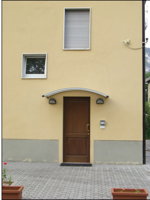
The Foyer and the entrance leading to the apartment
